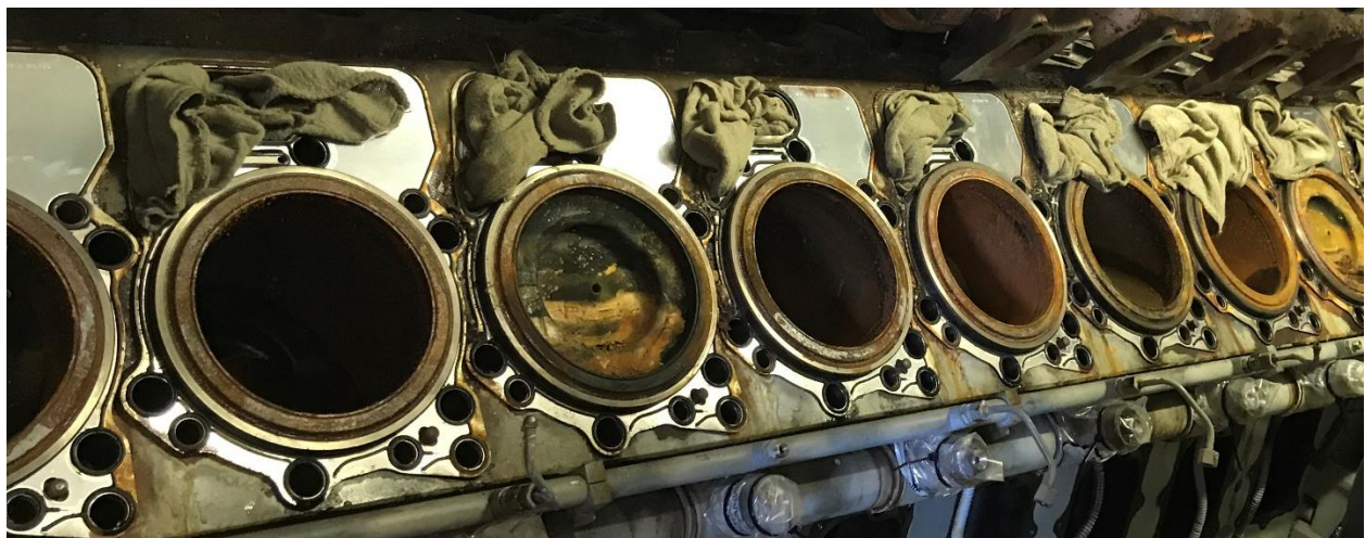
Figure 6 - Cylinder Liner and Piston Condition Observed During Disassembly
